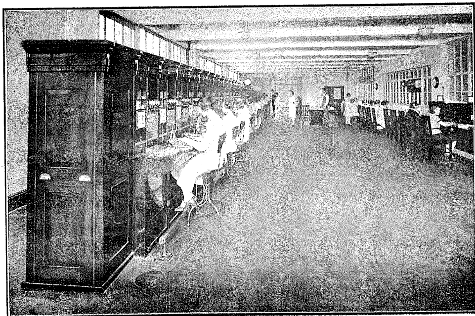
TRUNK SWITCH ROOM.
