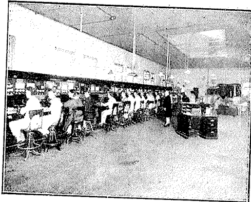
FORMER TRUNK SWITCHBOARD.
