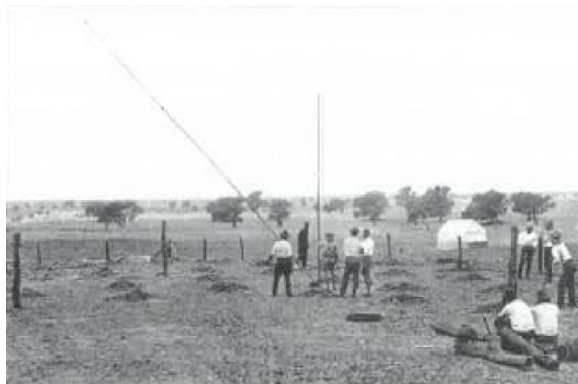
Installing and outpost antenna.
