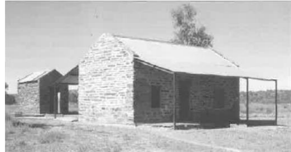
Restored Arltunga Police Station
