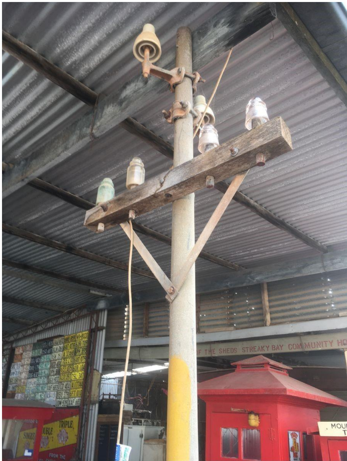
Siemen's Brothers tapered telegraph pole and insulators Streaky Bay Museum. 2022
