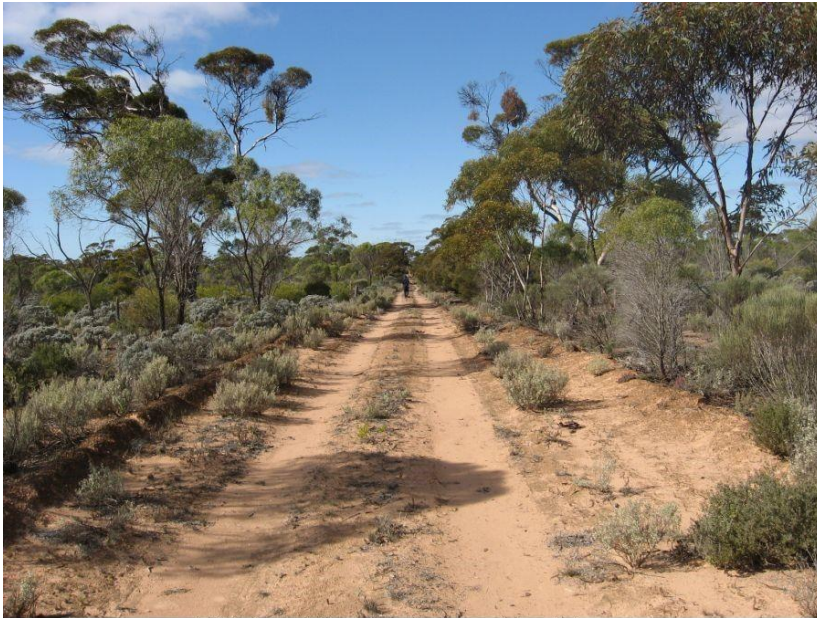
E W telegraph line where it crosses Eyre Highway Looking east. Modern underground cable down centre
