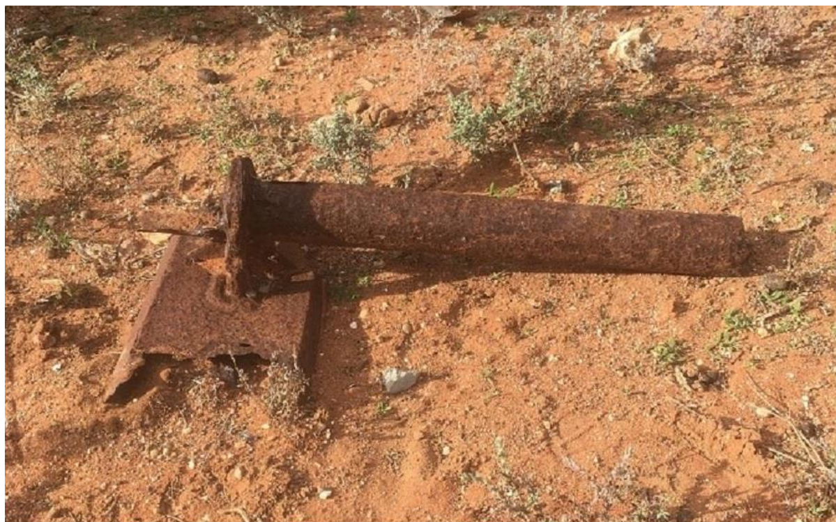
2021. Cook's house. Anchor plate attached to telegraph pole base section.
