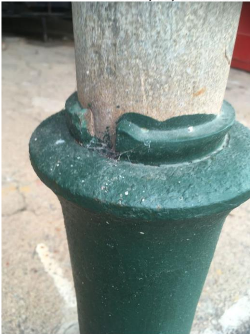
Siemen's Brothers tapered telegraph pole split wedge in base Streaky Bay Museum. 2022
