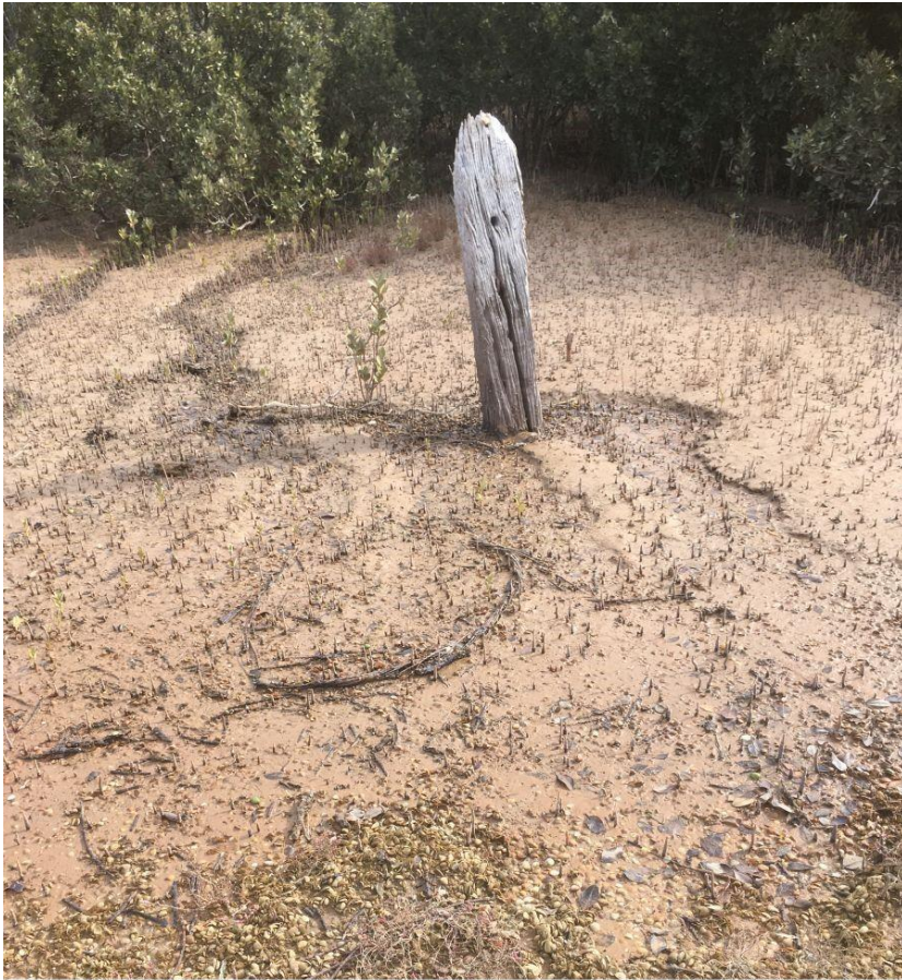
Pieces of cable at post 2
