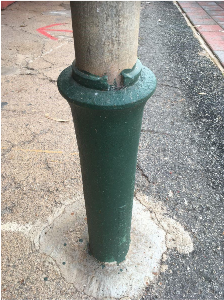
Siemen's Brothers tapered telegraph pole base and wedges Streaky Bay Museum. 2022
