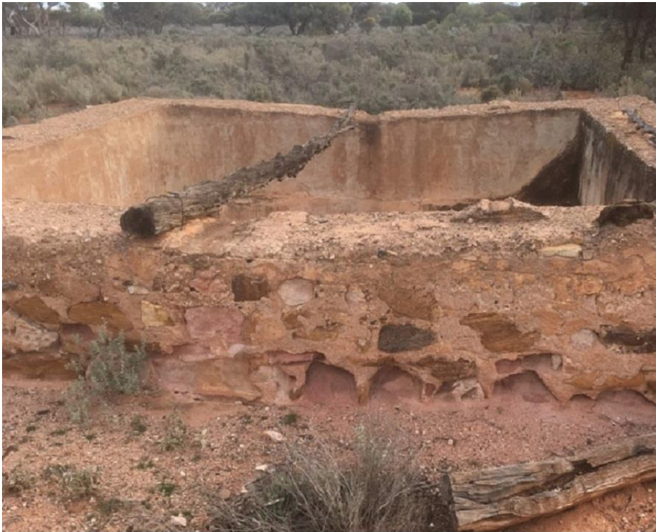
2021. Cook's house. Underground water tank.
